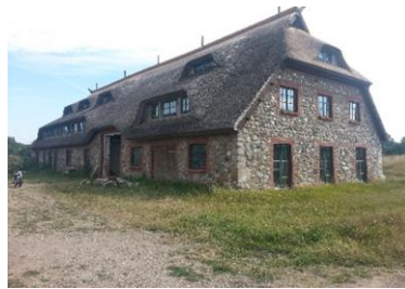
Country house in the Mutritz Country-park village of Speck. It is being sympathetically restored
